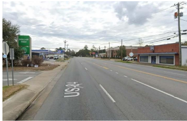
Quitman Commercial Corridor Character Area – Google Photo
